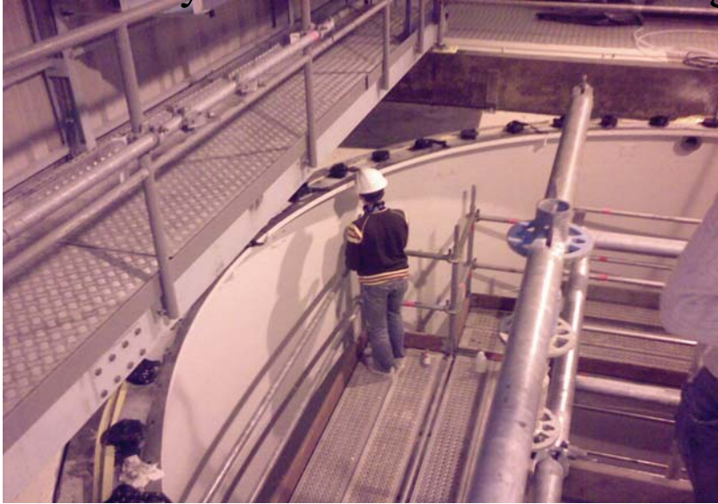
Inner veto PMT mounting
